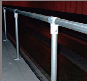
▲ Handrail in tunnel
