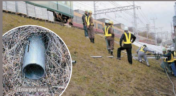
▲ Drain reinforcement pipe
