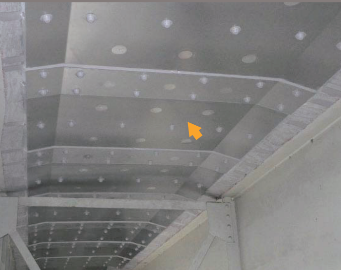
▲ Bridge reinforcing plate (steel plate adhesion method) ZAM® ZKS processing, ZAM Grout
