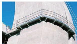
③ Inspection catwalk
