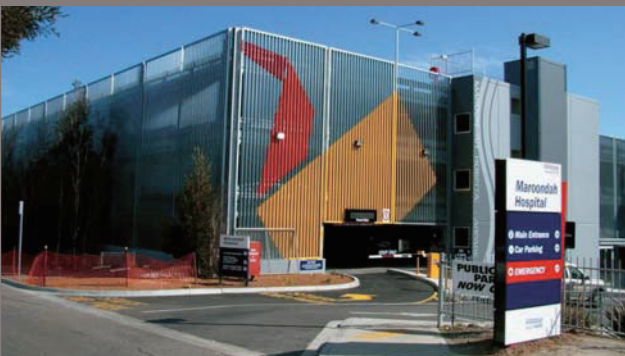
▲ Self-propelled multistory parking garage (distant view)
