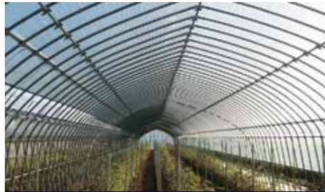
Green House Structure
