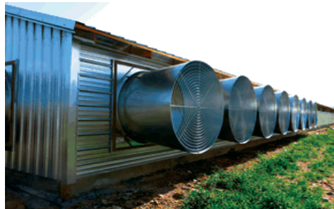
Animal Confinement Structure
